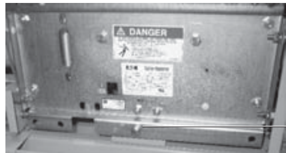
Figure 23. Remove Bolt-Down Hardware
