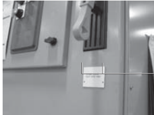
Figure 31. Drill Location for Emergency Entrance to Medium Voltage Compartment
