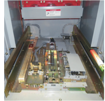
Installed BPI pan
