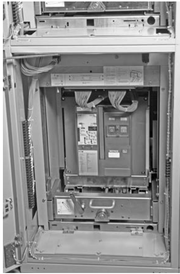
Circuit Breaker Compartment— Breaker in Connected Position
