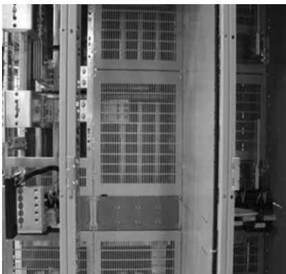
Optional Bus Compartment and Vertical Section Barriers
