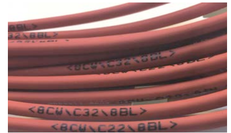
Control Wire Marking
