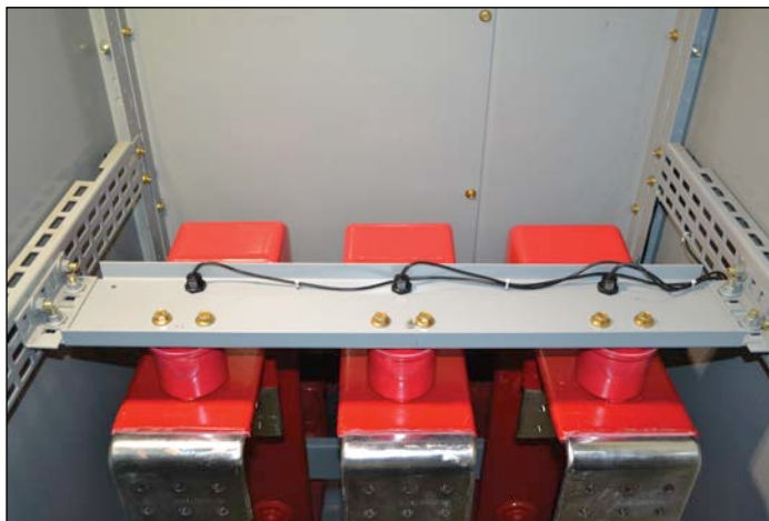
Figure 5.1-10. Typical Install for Continuous Thermal Monitoring Sensors
