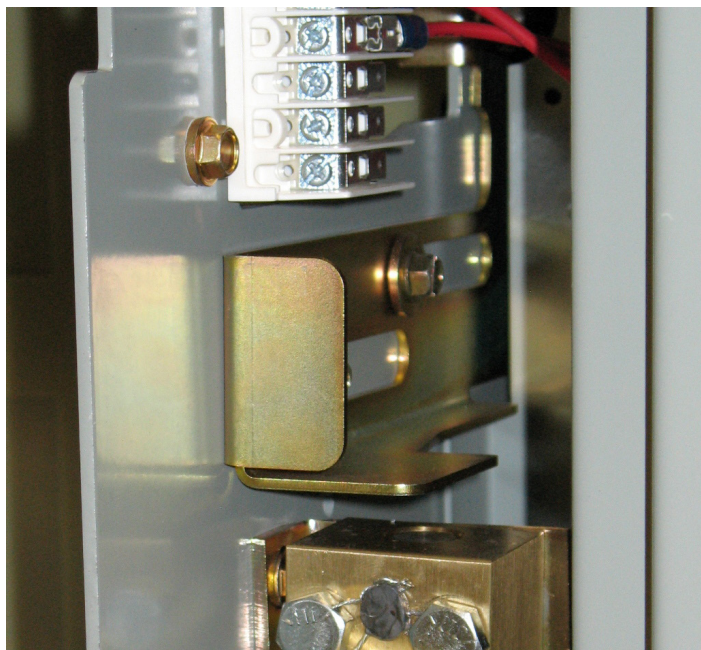
Figure 12. Magnum DS cell key interlock
