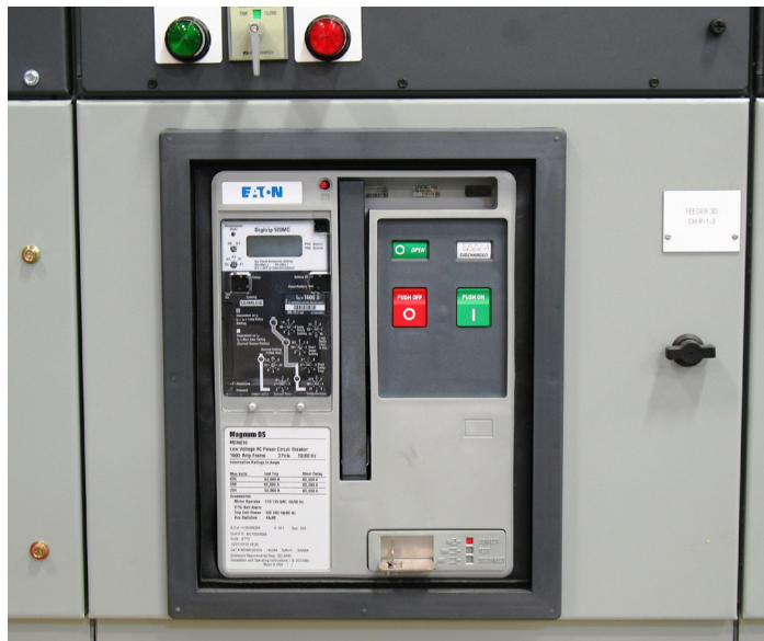
Figure 7. Magnum DS breaker in connected position
