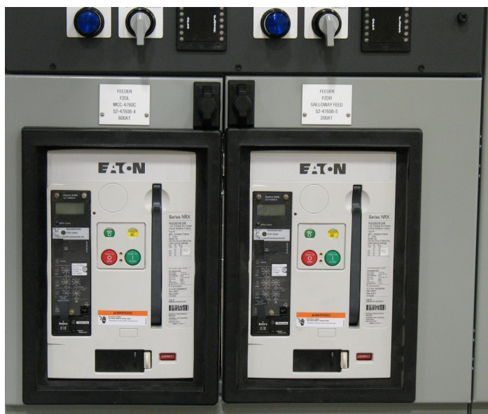
Figure 8. Series NRX breakers in connected position
