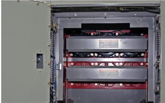
Figure 12. Automatic Shutters - Ring Type CTs with Shutters Closed and CT Barrier Removed.
