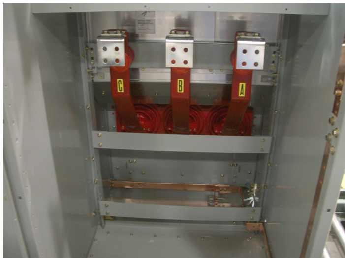
Figure 2. Ground Bus Installation.
