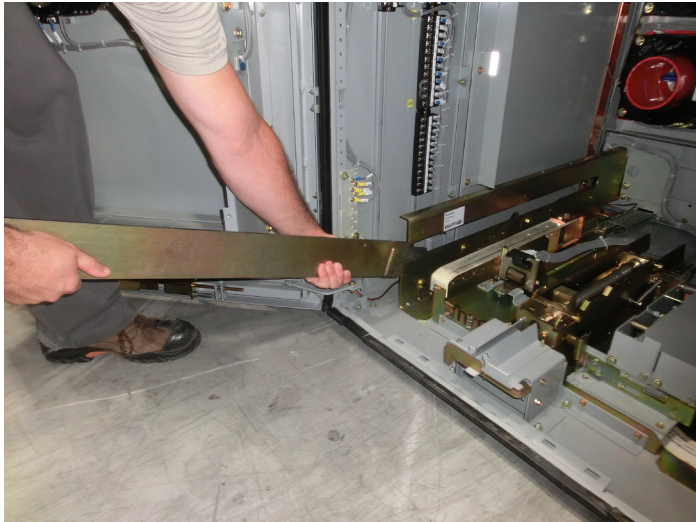
Figure 5. Insertion of the Drawout Extension Rails.
