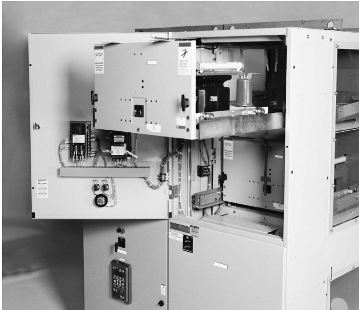
Figure 10. Drawout Drawer for Voltage Transformer on the Extension Rails.
