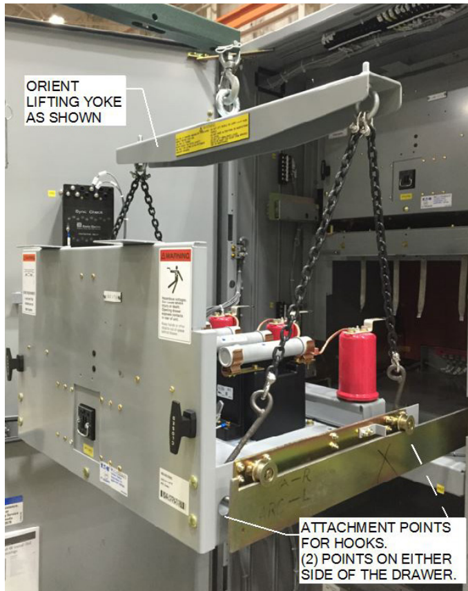
Figure 7. Lifting and Setting the Auxiliary onto the Extension Rails.
