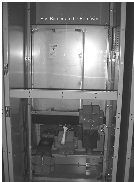
Figure 3. Main Bus Installations with Bus Barriers Installed. Viewed from the rear with the rear covers removed (typical 1-hi construction shown).
