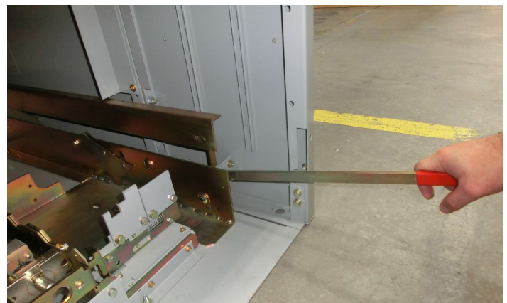
Figure 22. Hand Operation to Manually Open the Shutters
