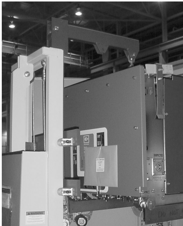
Figure 6. Lifting and Setting the Breaker in the Housing.
