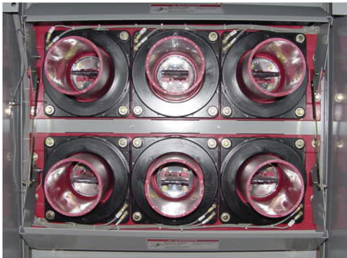
Figure 13. Automatic Shutters - Ring Type CTs with Shutters Open and CT Barrier Removed.
