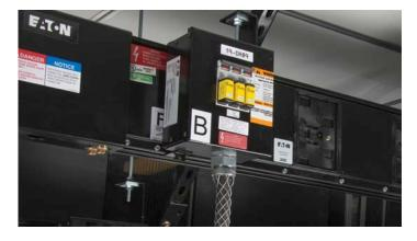
For ease of installation, Eaton's Pow-R-Bridge joint connections allow the busway sections to be joined to each other quickly without the use of special tools. Further, the busway sections are reusable and can be added, removed or repositioned per user requirements, allowing the company to make adjustments without the need to purchase additional units.
